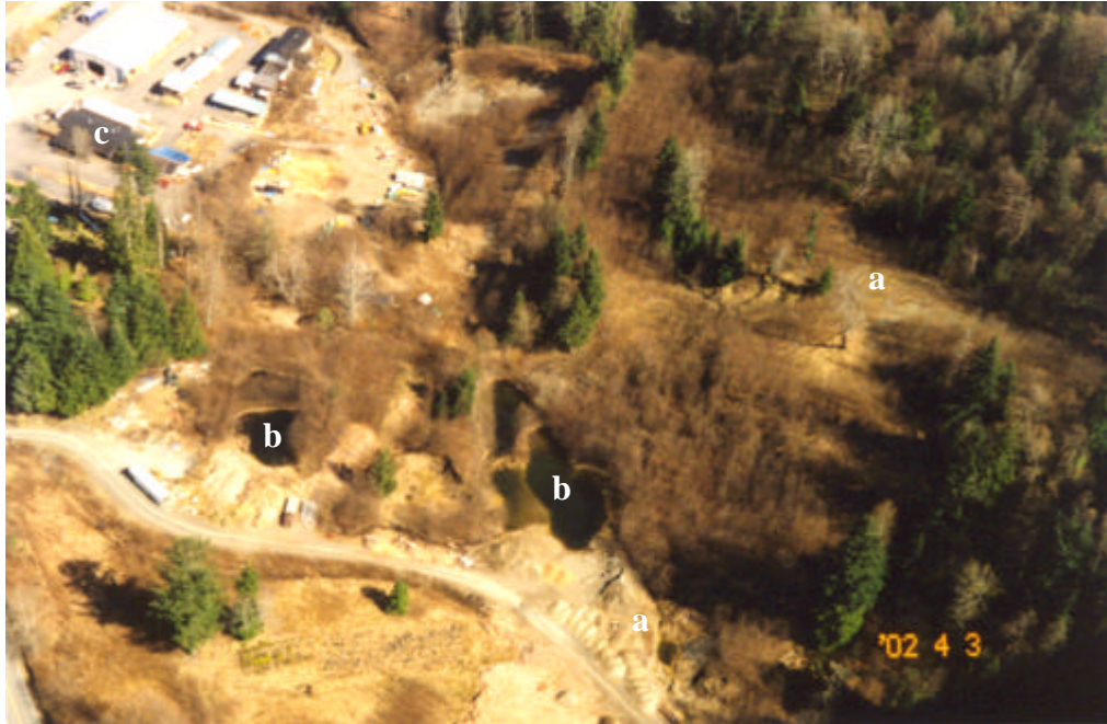
Photo 9. Site of former soil quarry (a) and sediment ponds (b) to west of lumberyard (c) in catchment 1-2 (Mac-Wha Creek). Grafton Rd is visible in lower left corner. 3-Apr-02
