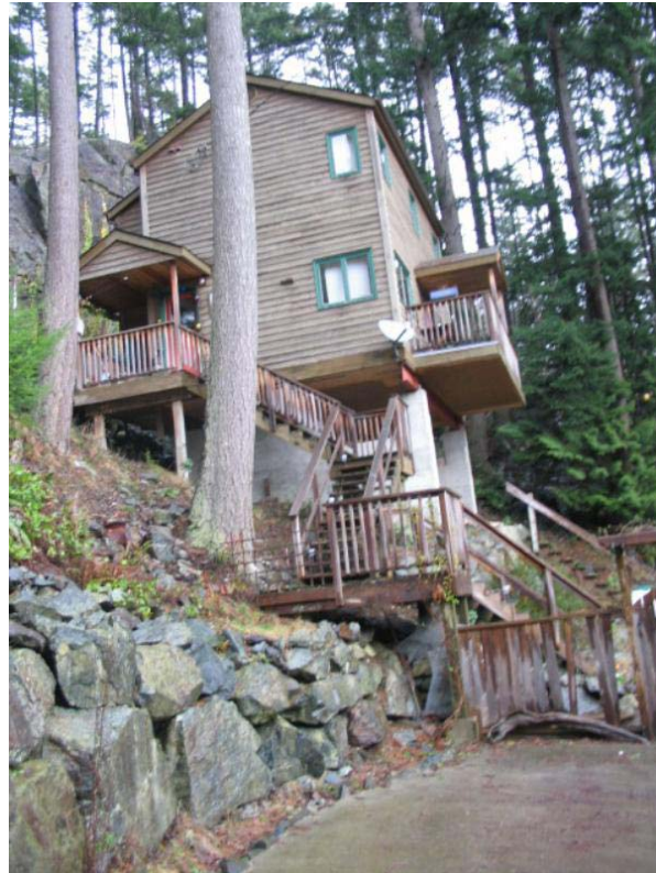
Figure 16. Example of home with wood siding and open decks and balconies.
