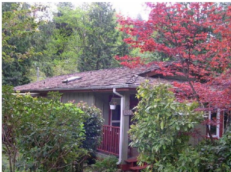
Figure 15. Photograph showing unrated roofing material present on many homes within the municipal wildland urban interface.
